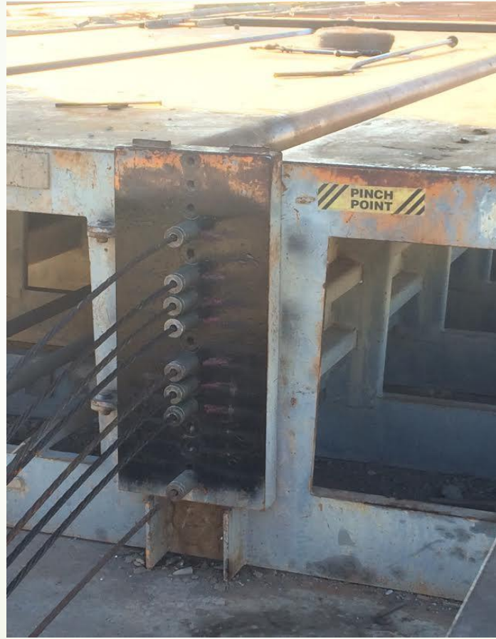
Figure 2: Casting Beds with Anchored Strands
